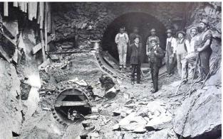
9.1. Just east of Austin Farm in Dorchester, Canterbury Brook was made to flow underground through the large conduit in the upper right, parallel to a smaller sewer line (lower left). *From Street Department Annual Report, 1906.*
